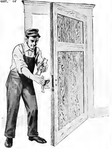
Your doors mortised for locks. No work for a chisel here. Simply slip the locks in place, drive the screws and the job is done.
